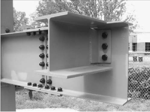
Figure 4-5. Shear Connection: Bolted-welded double-angle Girder B3 / Beam B3A
