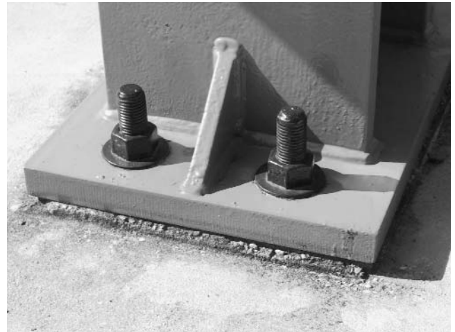
Figure 6-7. Column Connection: Base plate Foundation / Column C1
