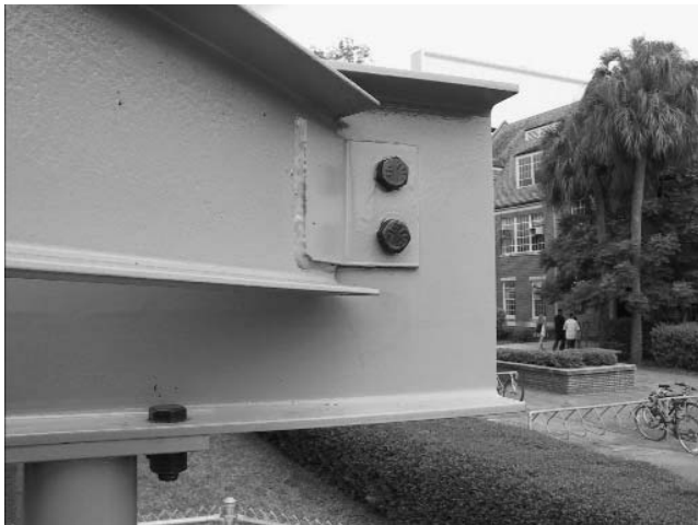
Figure 7-6. Misc. Connection: Bolted-welded bent-plate. Girder B5 / Beam B5A
