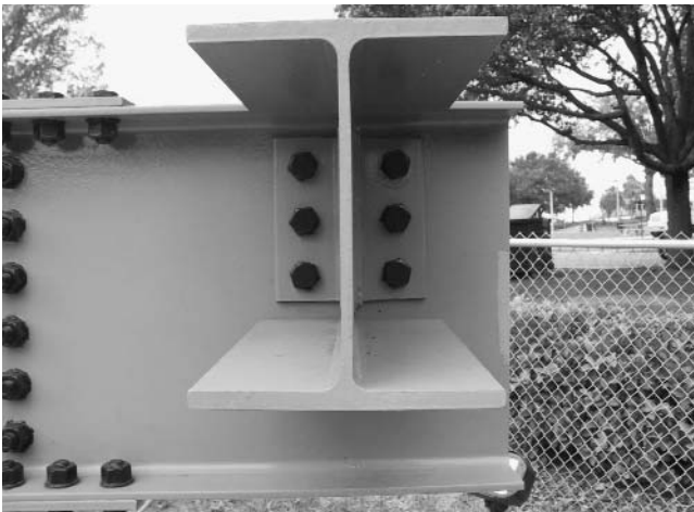
Figure 4-6. Shear Connection: Bolted-welded double-angle Girder B3 / Beam B3A
