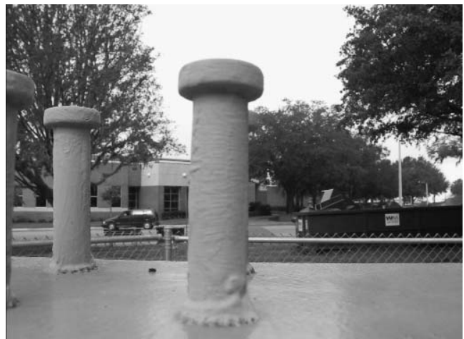
Figure 7-14. Misc Connections: Shear studs. Girder B1 / Shear Studs
