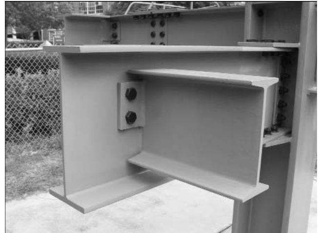
Figure 4-24. Shear Connection: Bolted shear end-plate Girder B2 / Beam B2A
