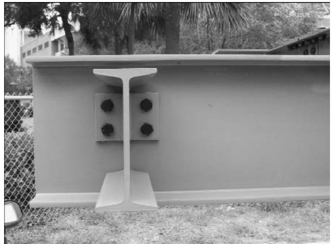
Figure 4-22. Shear Connection: Bolted shear end-plate Girder B2 / Beam B2A
