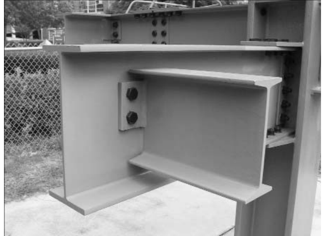
Figure 4-21. Shear Connection: Bolted shear end-plate Girder B2 / Beam B2A
