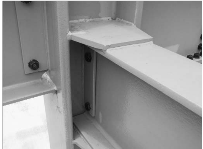
Figure 5-4. Moment Connection: Welded flange plates Column C1 / Girder B4
