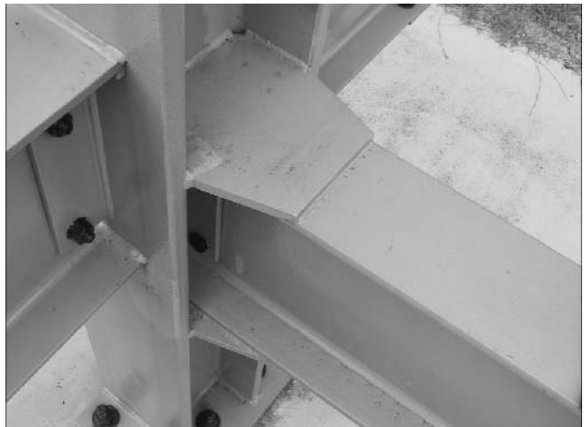
Figure 5-5. Moment Connection: Welded flange plates Column C1 / Girder B4
