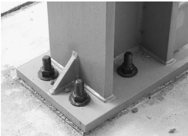
Figure 6-6. Column Connection: Base Plate Foundation / Column C1
