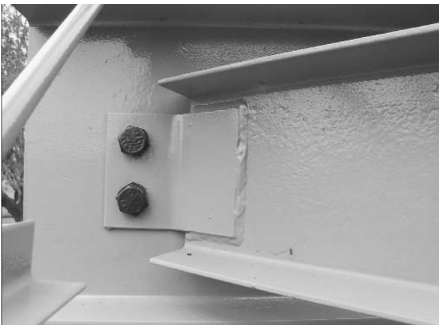
Figure 7-7. Misc. Connection: Bolted-welded bent-plate. Girder B5 / Beam B5A
