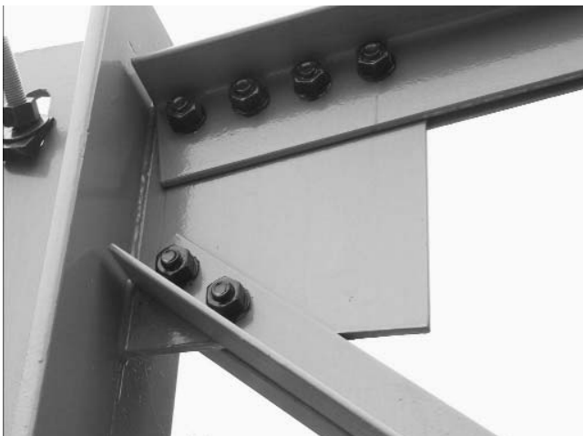
Figure 7-17. Misc. Connection: Truss Column C2 / Truss B7
