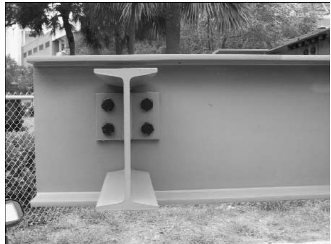
Figure 4-25. Shear Connection: Bolted shear end-plate Girder B2 / Beam B2A
