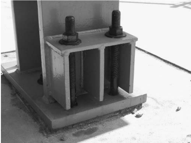
Figure 6-4. Column Connection: Base plate Foundation / Column C1
