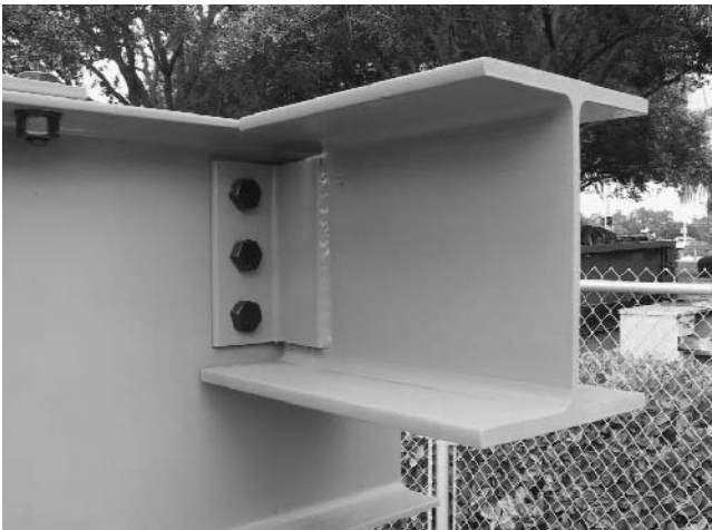
Figure 4-7. Shear Connection: Bolted-welded double-angle Girder B3 / Beam B3A
