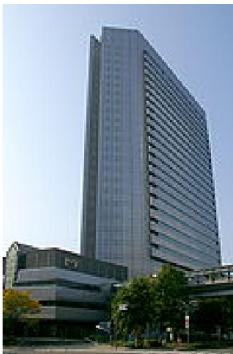
The Panasonic IMP Building in Osaka , Japan
